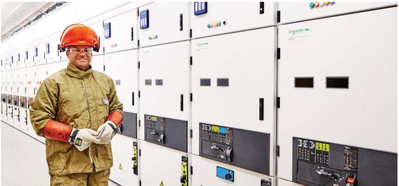
Kununurra back-up power station.
