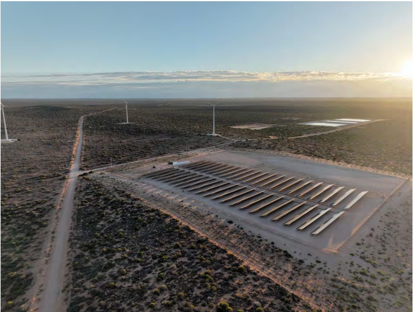
Denham hydrogen demonstration plant - solar farm
